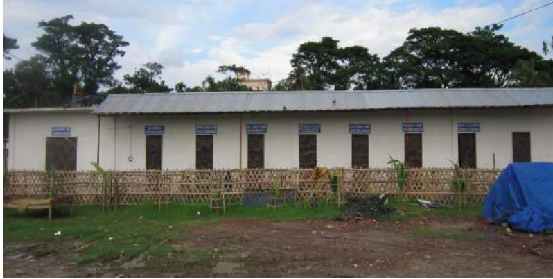
(a) Storage facility of hazardous wastes and other materials
